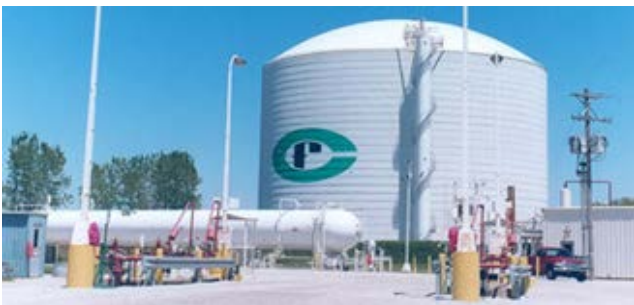
Figure 6. “Atmospheric” refrigerated liquid anhydrous ammonia (NH 3 ) tank stores 190,000 MWh as 30,000 MT of NH 3 fuel. Total capital cost ~$ 15M; ~ $ 0.10 / kWh
